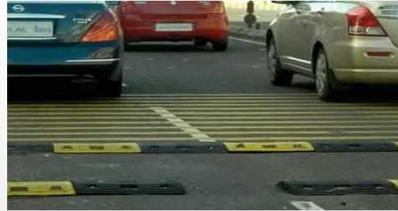
Height Constraint Barrier Speed breakers with missing Sections
