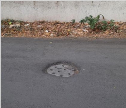
Manhole Below Road Level
